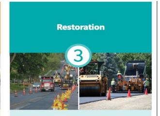
When all underground construction work is completed, we will restore the affected areas. In general, surface restoration is done to meet the pre-construction conditions. For in-road construction, typically, a section of the pavement will be milled and paved during this process.
