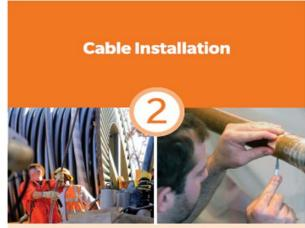
Cable installation takes place after the duct bank and manholes are installed. The cable is pulled from a reel between manholes and structures along the route.
