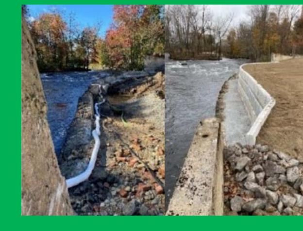
One of the project's greatest challenges was the repair or replacement of a 100foot section of a retaining wall that had collapsed after years of erosive deterioration from the adjacent Willimantic River. With the escalation of drastic weather events in the region in recent years, a new section of retaining wall was installed to protect the site from severe flooding events.
